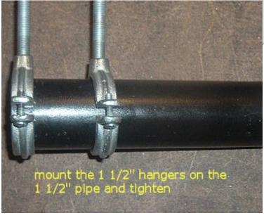
STEP 4 – Mount the 1 1/2" on the 1 1/2" pipe and tighten.
